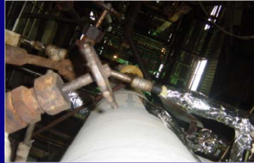
Looking Up the Column
